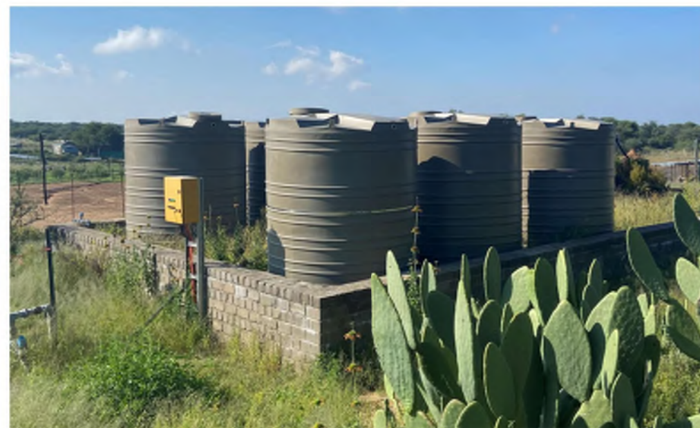
PI-i: Example Storage Tanks reserve water tanks at CCF Namibia facilities, several 10,000-liter reserve water tanks will ensure there is not a water shortage for multiple days' activities.
