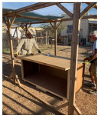
IN-e: CCF volunteers building SH1
