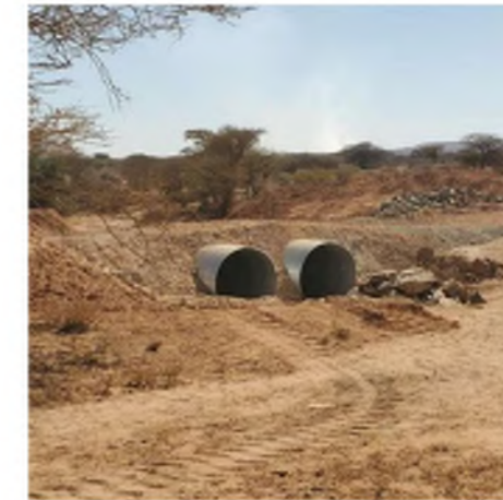
PI-a: Wadi Crossing - Pipe Culvert large pipe culvert along pipeline road
