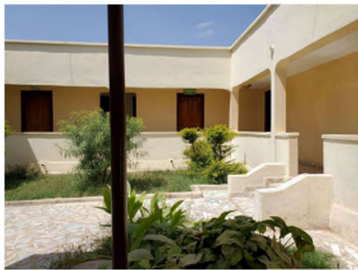
PB-i: courtyard office, Ministry of Environment and Rural Development
