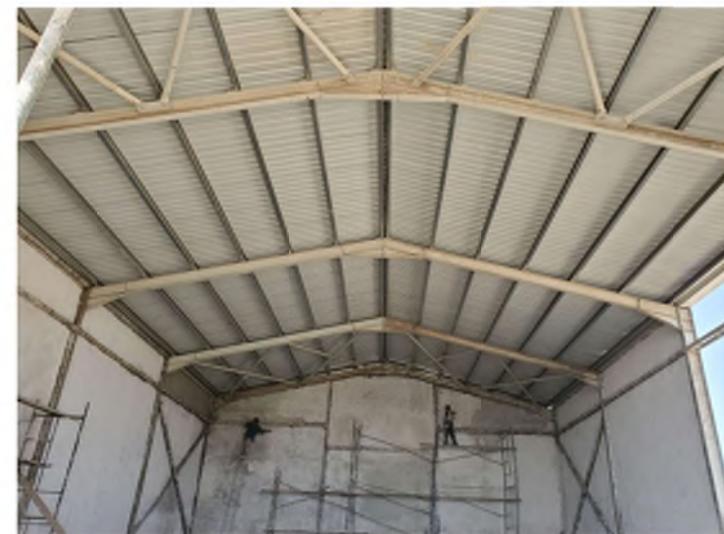
PB-k: steel construction in Hargeisa
