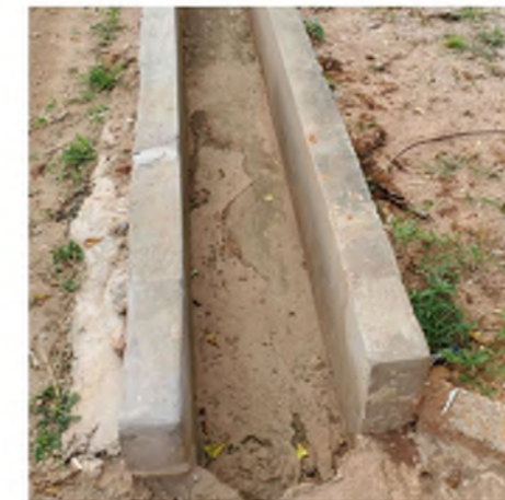
PI-c: Channel concrete water channel for water diversion
