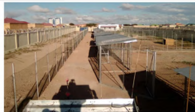
IN-j: SH2 enclosures near completion
